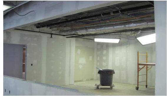
Drywall work at the conference room
